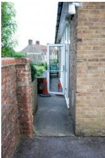
Side access to disabled entrance to left of main entrance
